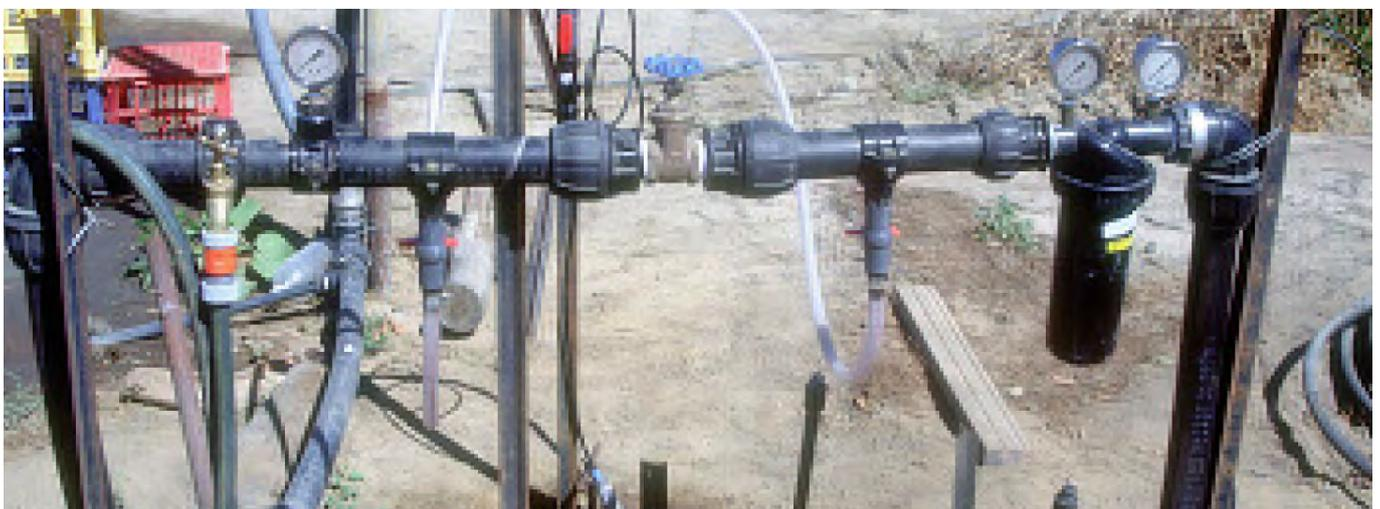
*A simple manifold set up with a venturi injector, pressure gauges and a valve causing the required pressure drop.*
